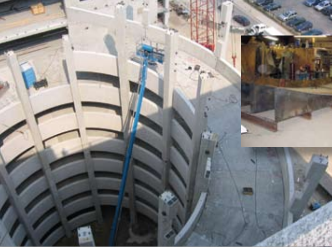
Precasters constructed the double-helix ramp at the center of the structure by creating custom forms that turned and sloped in precise configurations.
