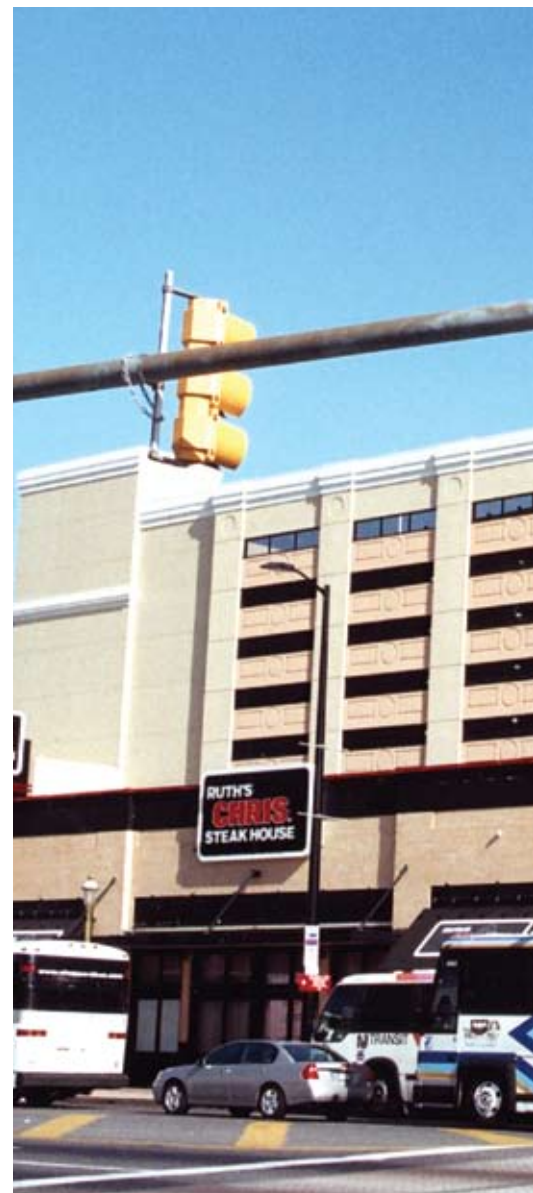
Using two crews and a total-precast concrete system to construct the new 1.1 million ft 2 parking structure at Bally Caesar's Casino in Atlantic City, N.J., cut construction time by about 40%.
