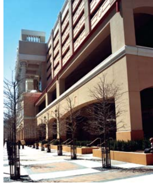
Using two crews and a total-precast concrete system to construct the new 1.1 million ft 2 parking structure at Bally Caesar's Casino in Atlantic City, N.J., cut construction time by about 40%.
